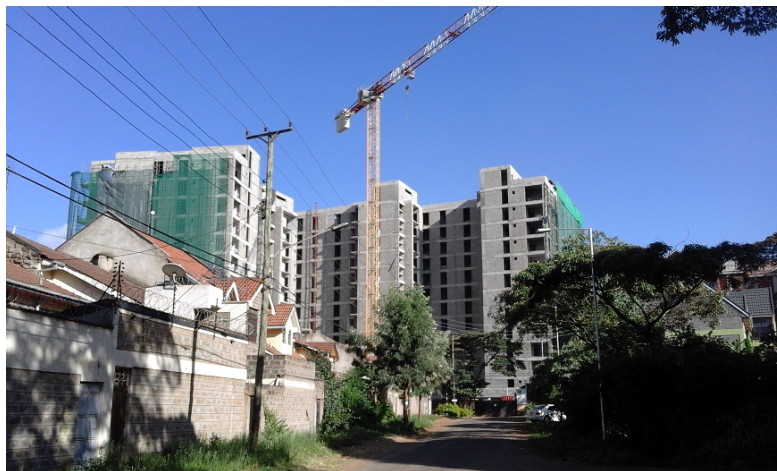
Figure 1. Signature Apartment, a high-rise apartment block under construction in Kileleshwa (author, 2015)
